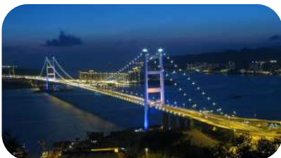
Tsing Ma Bridge
